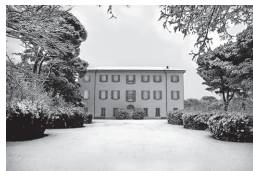
pp. 58-61 Villa Bellaria, Furla headquarters in San Lazzaro di Savena (BO)
